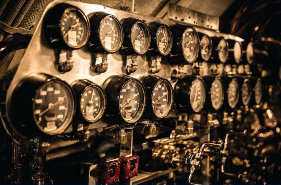
(Top) Engine room gauge panel. (Bottom) Ohio-class submarine transiting in open ocean.
