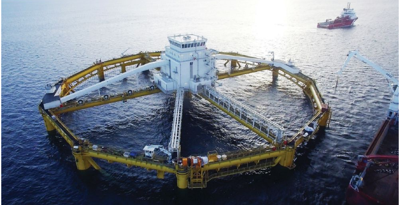
(Above) Ocean Farm 1 lowered into the water. (Credit: SalMar) (Below) Sensor installation on Ocean Farm 1. Sixteen high-precision fiber-optic sensors from Light Structures' SENSFIB technology range have been installed on site. (Credit: SalMar)
