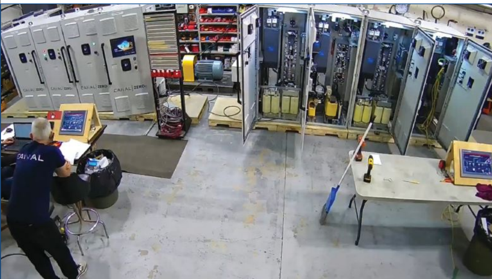
Work in progress building out the electrical system that now powers the ferry. (Credit: Canal Marine and Industrial)
