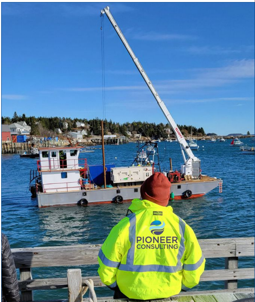
Isle au Haut installed its first subsea telecommunications in November 2024. The 10-km submarine cable now connects Isle au Haut to Stonington on Deer Isle, which has terrestrial connections to the U.S. mainland. (Credit: Donna Hopkins, Isle au Haut Broadband Committee)
